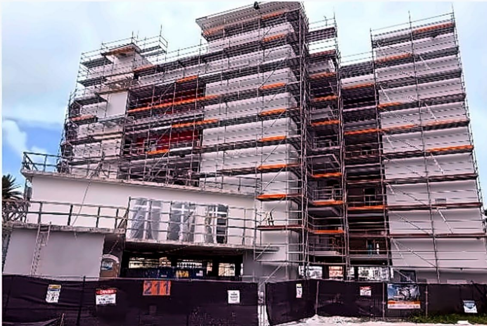
SITE • CONSTRUCTION PROGRESS
